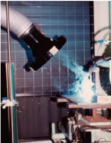
Local Exhaust Ventilation.
