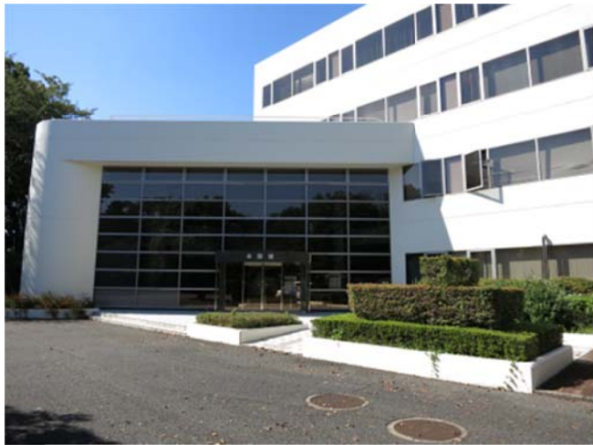
Entrance of main Building.
