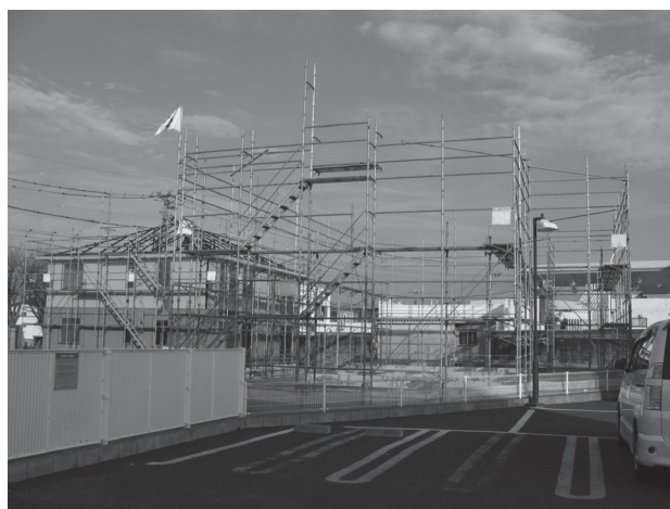
Fig. 10. Scaffolds erected by the preceding scaffold construction method.
