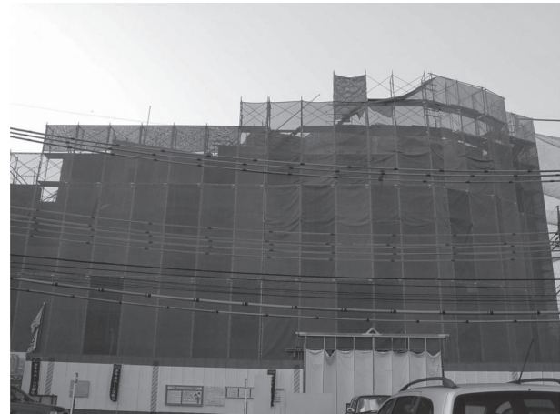
Fig. 2. Scaffolds covered with scaffold sheeting.
