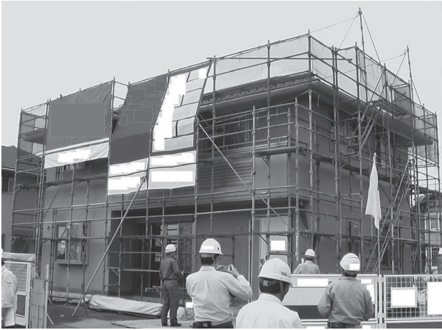
Fig. 11. A house constructed by the preceding scaffold construction method.
