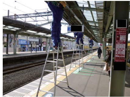
Figure 7. Roof repair work with safety features Figure 8. Unsafe usage of stepladders
