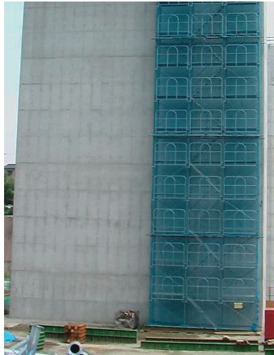
Figure 12. Prefabricated scaffolds erected by the Advanced Guardrail Installation Method
