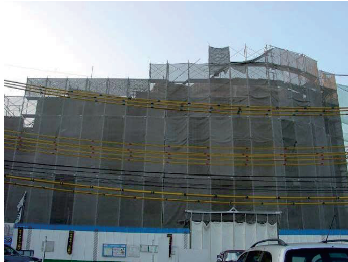
Figure 1. Scaffolds covered with sheeting
