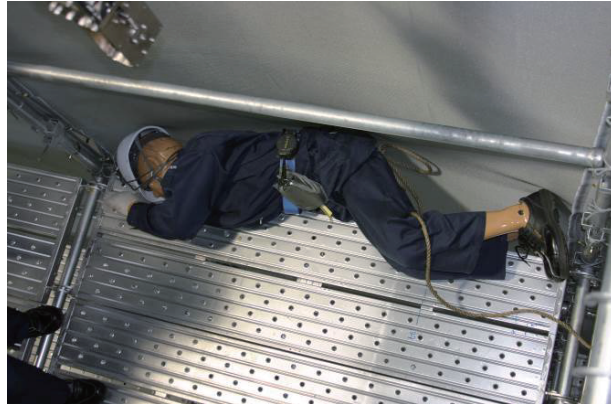
Figure 2. A worker making room for movement by pushing the sheeting
