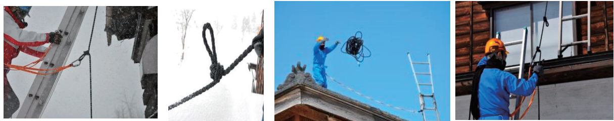
Figure 4. (Left) Simple yet effective: loop on vertical lifeline. (Right) Deploying the lifeline.
