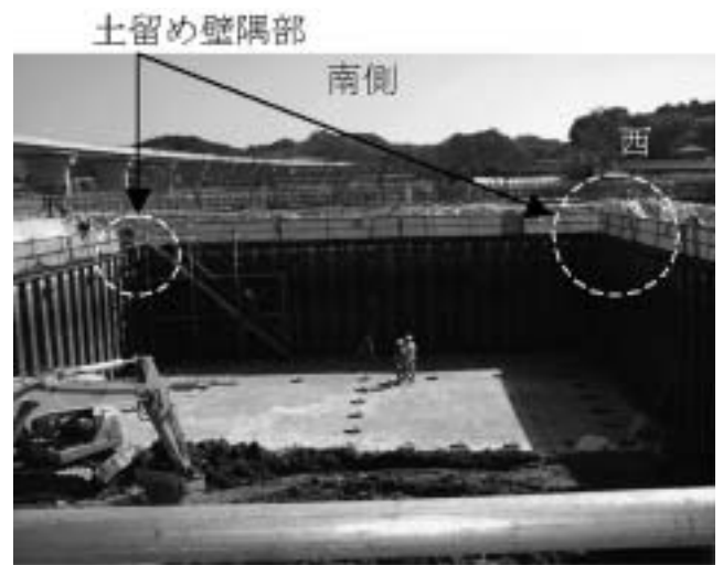
Photo. 6 View of the construction site. 現場全景
