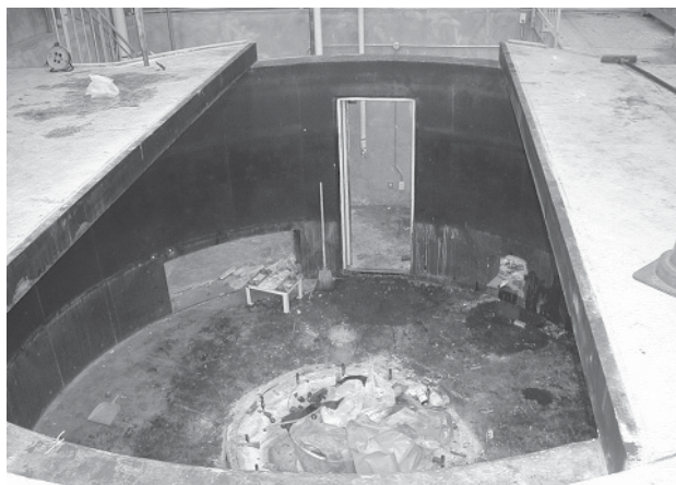
Photo 12 Dismantle NIIS Mark-1 Centrifuge. 旧遠心模型実験装置の撤去
