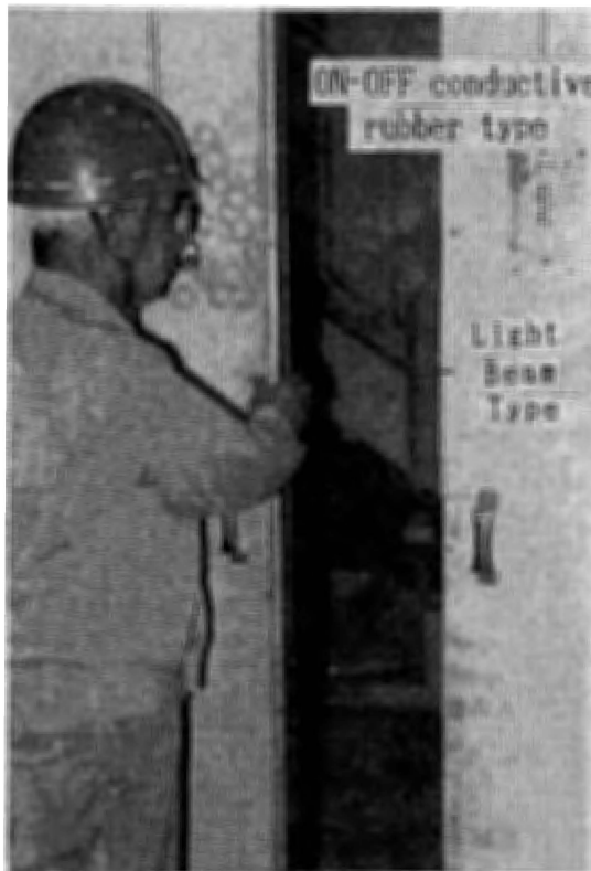
Photo 7.2 Safety edge of light-beam type and conductive rubber type 光線式と導電ゴム式のセーフティ・エッジ
