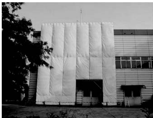
Photo 1 Scaffolds set alongside the building.
