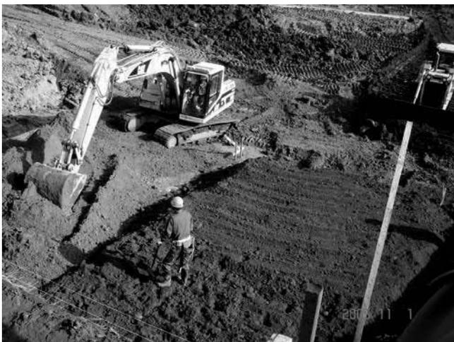
Photo 4 Spreading soils.
