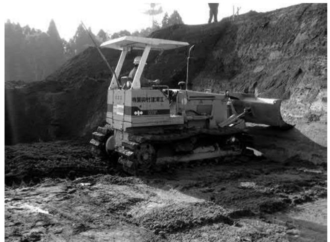
Photo 5 Bulldozer using roller compaction.
